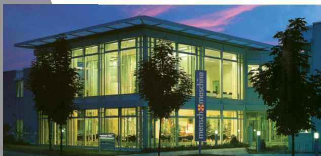
The new M+M solar power plant in Wessling
